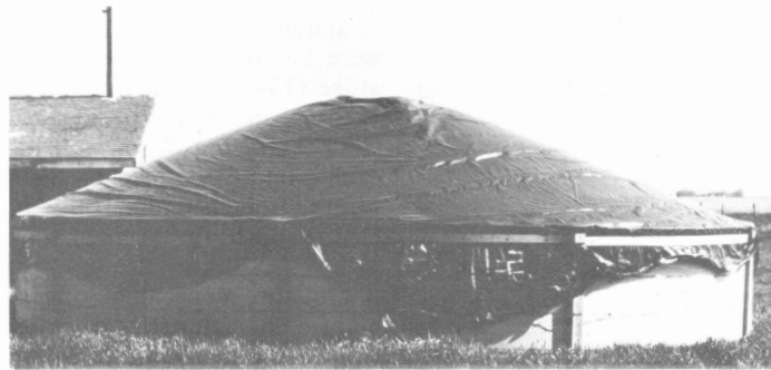
Figure 1. Temporary grain bin covered with polyethylene sheet (bin no. 11, Table I).
