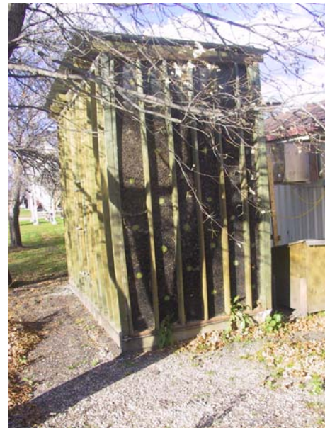
Fig. 3. Exit face of the experimental biofilter (Side A) constructed adjacent to a hog barn at the university research farm. A plywood duct channeled the air from the barn to the biofilter.
