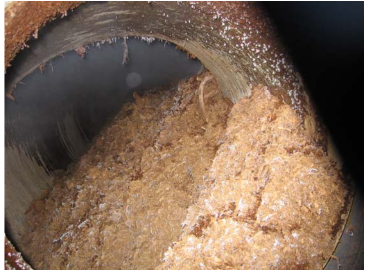
Photo 5, December 14, 2005: Interior view from the exit opening, exterior temperature of -25^{\circ}\text{C} .
