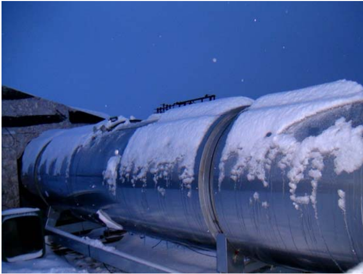
Photo 4, December 16, 2005: Exterior installation.
