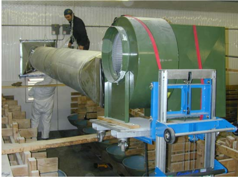
Figure 1. Installation of the standardised conduit inside one room.
