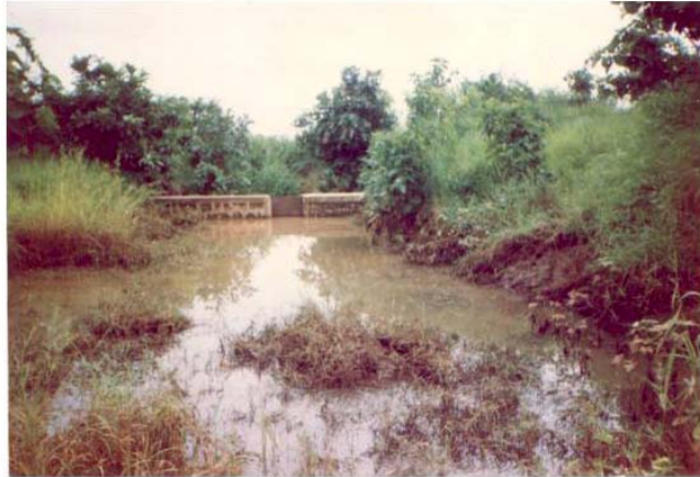
Cement plug CP1 with impounded water
