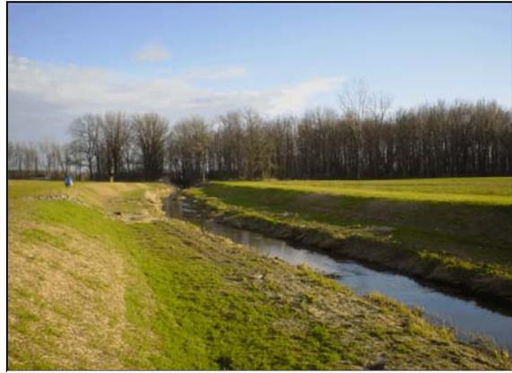
Figure 2. A constructed two-stage channel in Hillsdale County, Michigan.
