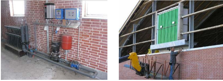
Figure A1. The frequency-regulated circulation pump and GEO control (left) and the heat exchanger (right).
