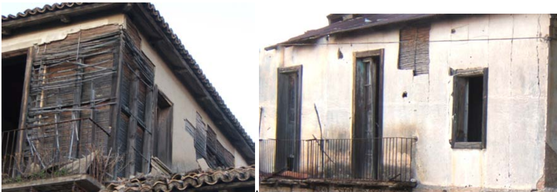
Figure 2. Rural buildings in the south of Italy with external walls panelled with Arundo donax .
