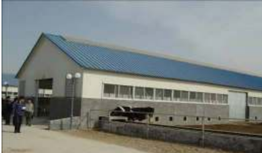
Fig 2. Double sloped cattle house in wet-hot area (electrical window system on the top)
