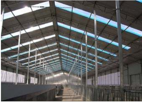
Fig 3. Cattle house in dry-cold area (lighting belt on the top)
