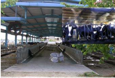
Fig 1. Opened cattle house in dry-hot area (fan and spray cooling)
