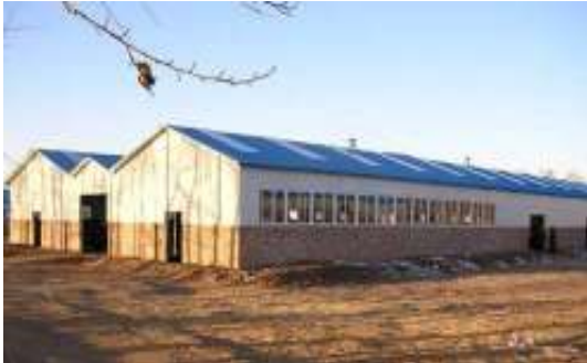
Fig 4. Multi-span cattle house in wet-cold area (lighting belt and forced aerator on the top)
